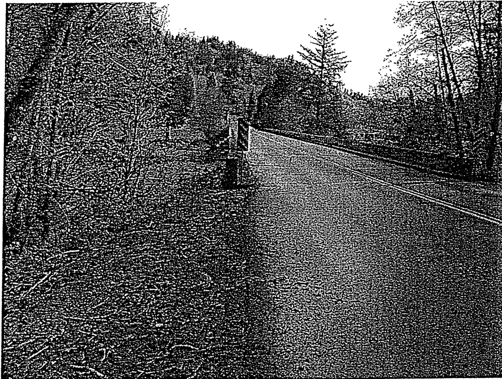
SW Corner Reiersen Bridge
